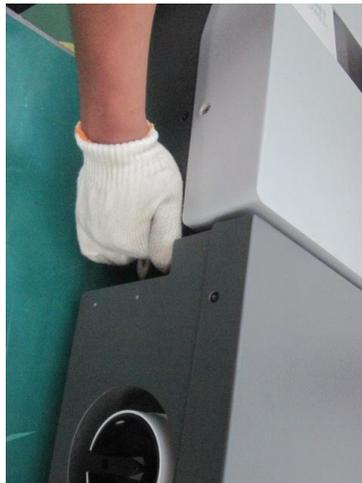
Figure 3-7b Mounting inverter on the bracket
