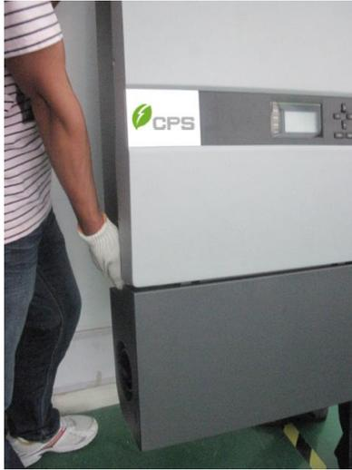
Figure 3-7c Mounting inverter on the bracket
